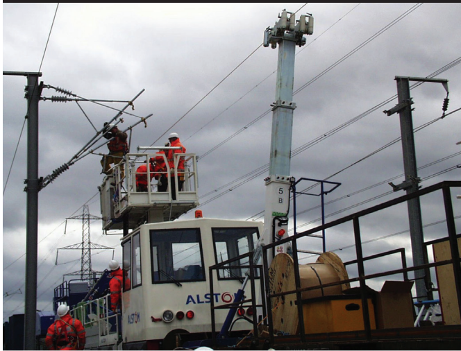
Translating and Swinging Telescopic Mast for final positioning (opt. 131.1)
